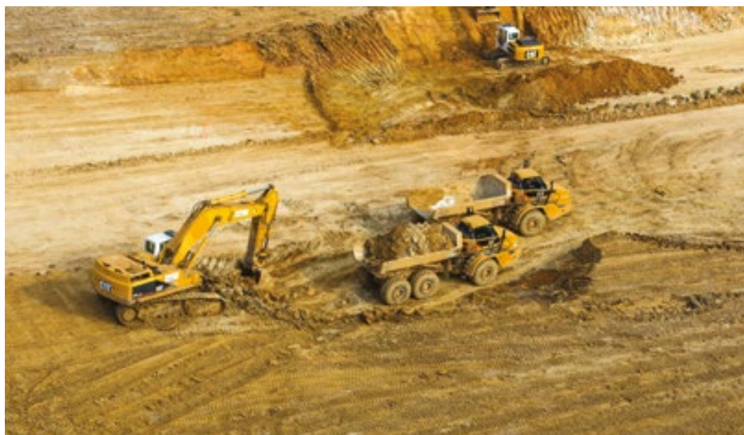
Terrassements, Sorigny, Indre-et-Loire, 2013
