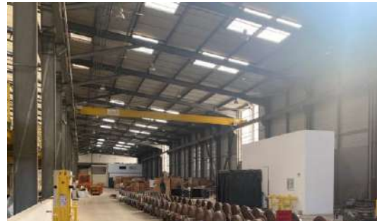
Maintenance preventive et corrective
